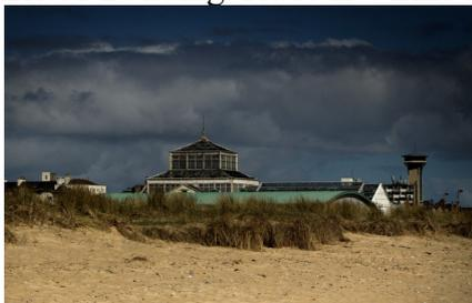
South, its condition is stated as being poor. Built with Cast iron components which are corroding because of excess moisture leaking into the structure. It is located within the conservation area that includes the seafront.
